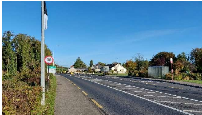
Existing N3 National Primary Road
